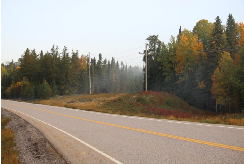
Photograph 15: View of Station 2 along Highway 101 (September 26, 2023).
