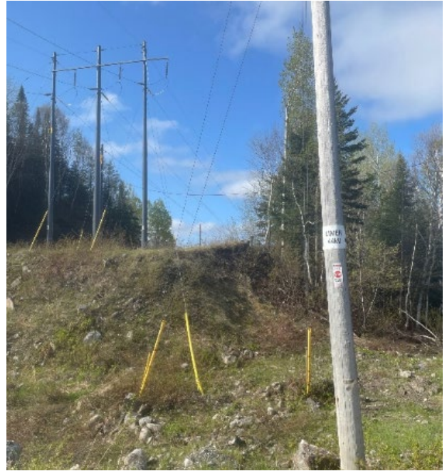
Photo 3: Example of triple pole group for support at turns or dead ends
