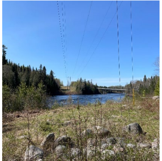
Photo 4: Example of span across water course
