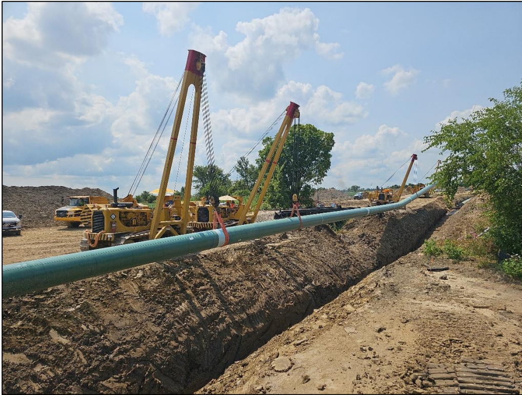
3. Pipeline lowering in near a watercourse crossing.
