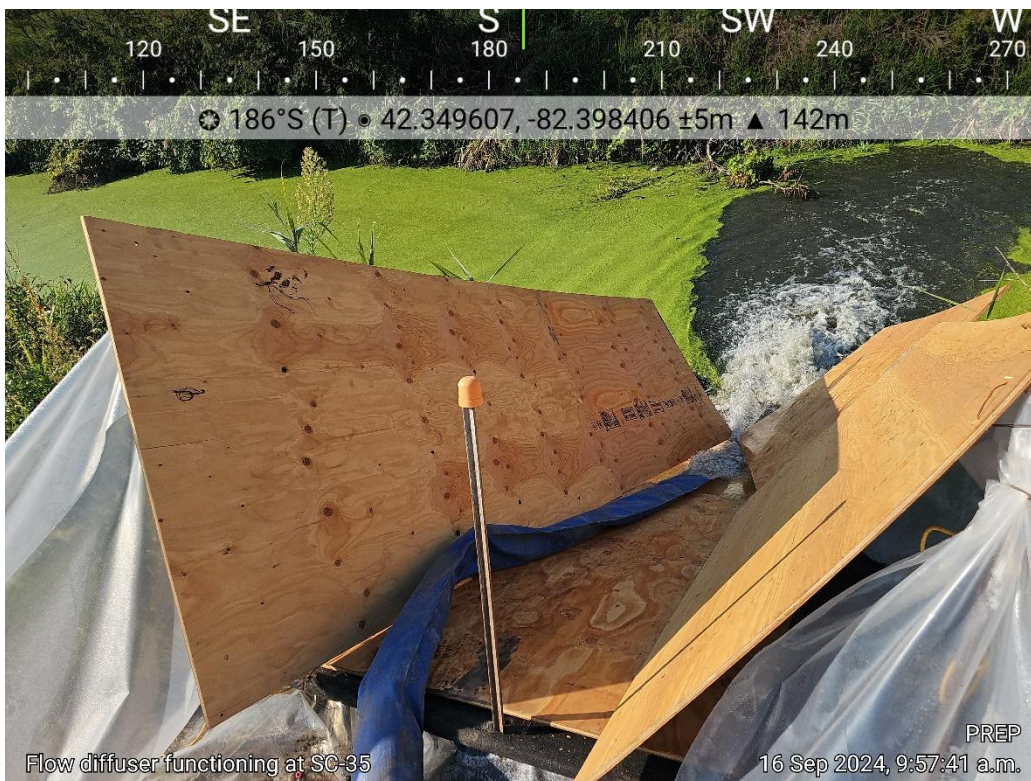
10. Flow diffuser being utilized during hydrostatic test water discharge.
