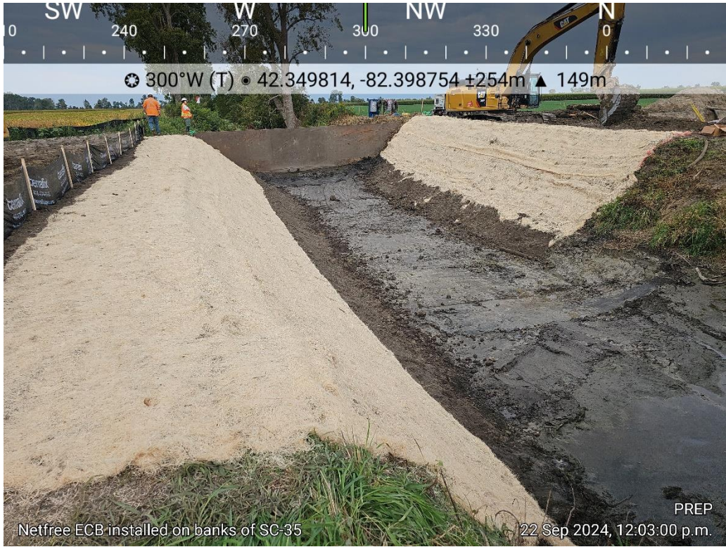
7. Watercourse crossing restoration with erosion controls in place.
