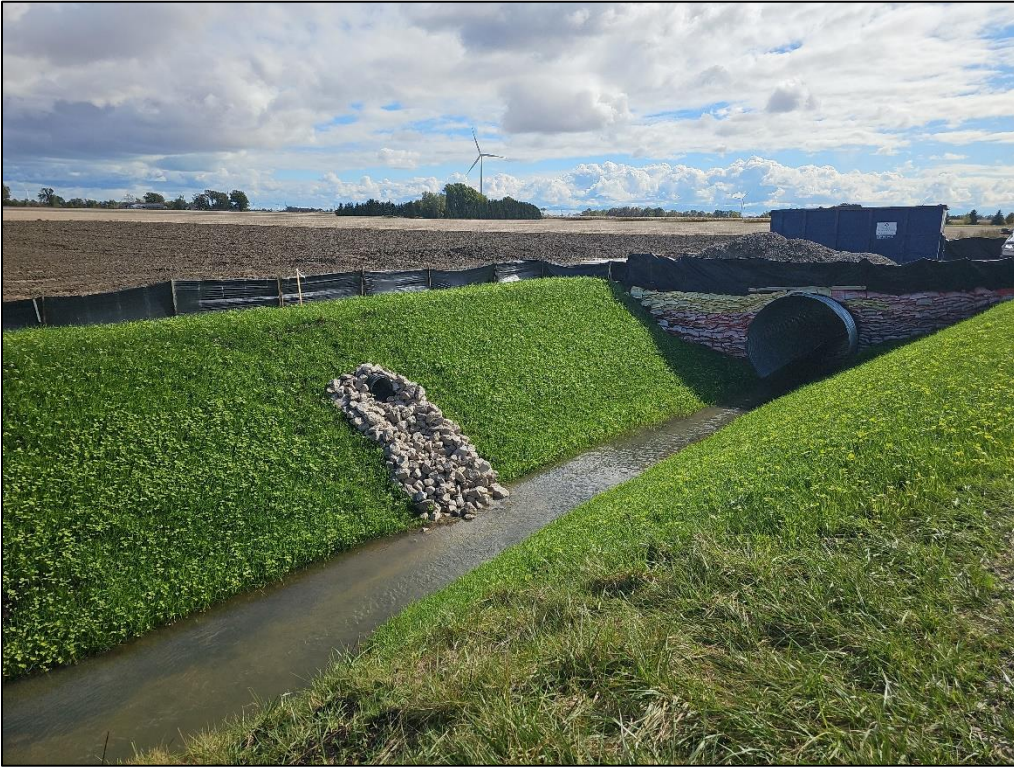
1. Restoration of open cut pipeline watercourse crossing.
