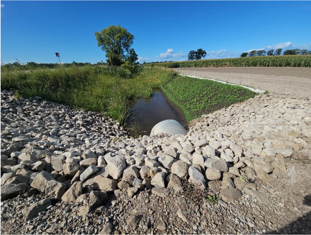
13. Stream Crossing #33 after restoration.
