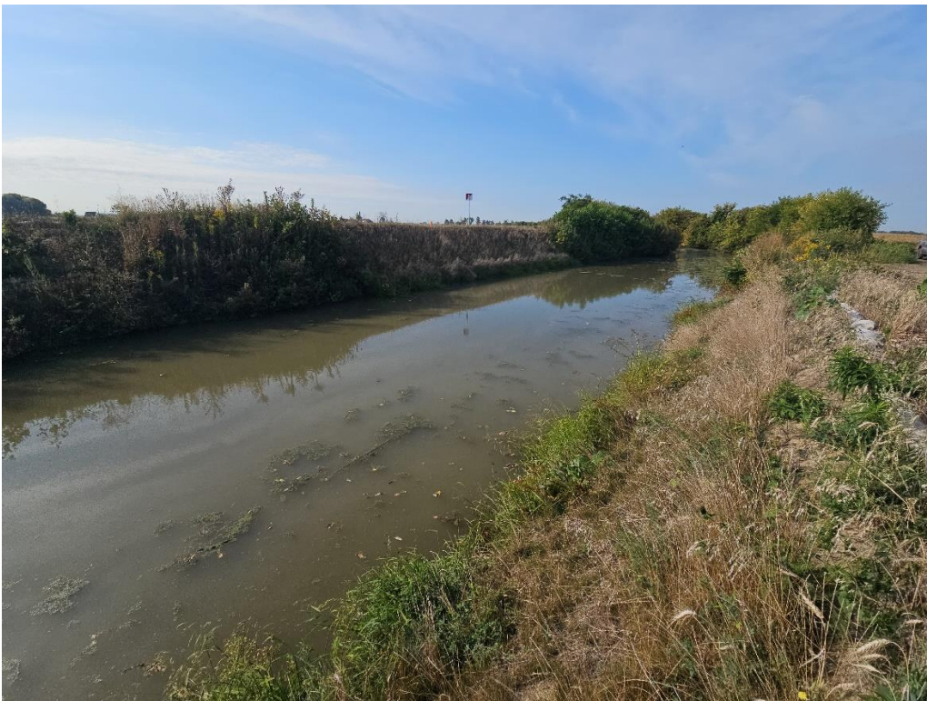
12. Stream Crossing #25 after restoration.
