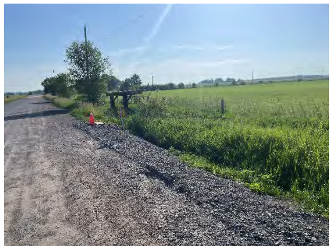
Photo 42: Regraded and back-filled ROW along Mcguinty Road (June 30, 2025).
