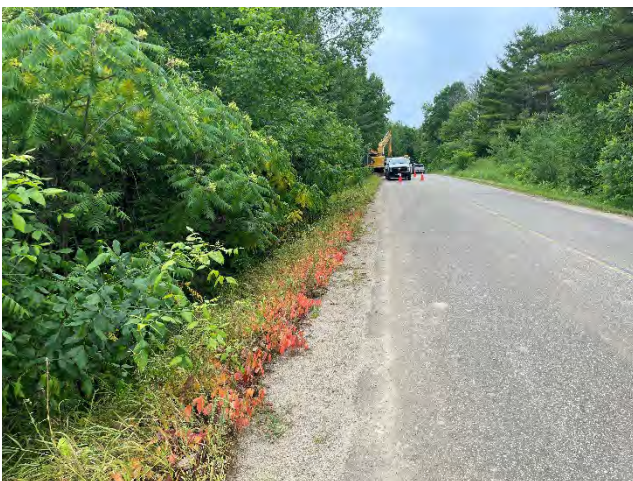
Photo 41: Existing conditions on Mcgaghran Road after spraying of poison ivy (June 30, 2025).
