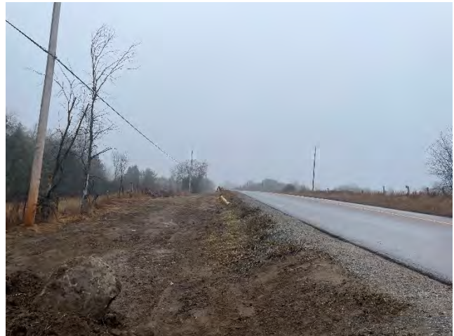
Photo 70: Restored road embankment on Letts Cemetery Road, north of Snodrifters Road (November 26, 2025).
