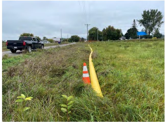
Photo 2: Pipeline stringing activities on Micksburg Road ROW. (September 23, 2024).
