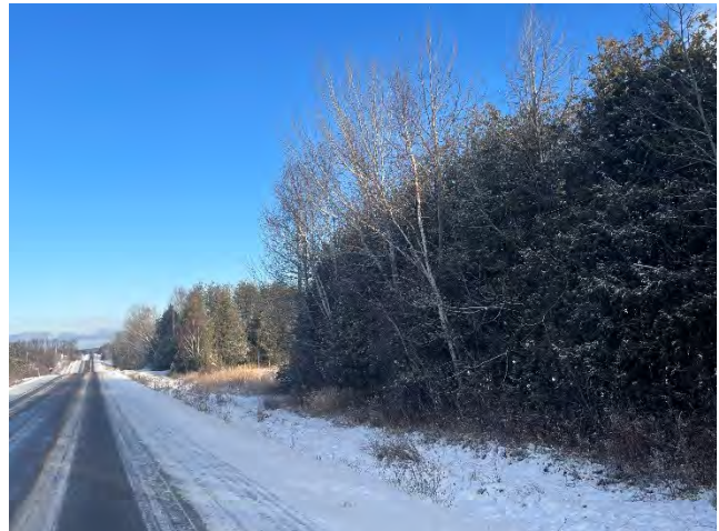
Photo 72: Completed restoration at corner of Cold Creek Road and Letts Cemetery Road (December 2, 2025).
