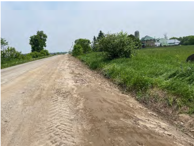
Photo 35: Restoration completed at Mcquinty Road, east of Micksburg Road (June 6, 2025).
