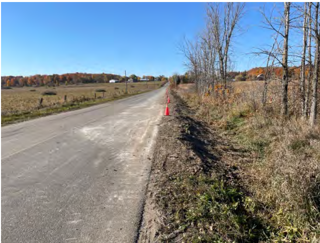
Photo 9: Partially reclaimed embankment along Mcgaghran Road (October 21, 2024).
