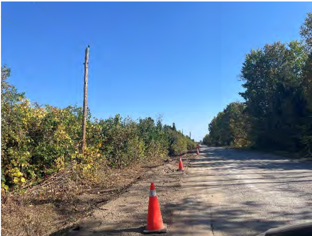
Photo 57: Restoration completed on Cold Creek Road, west of Bulger Road (October 3, 2025).
