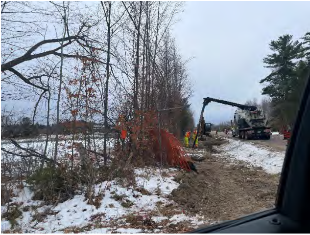
Photo 67: Partially restored ROW along Letts Cemetery Road (November 19, 2025).
