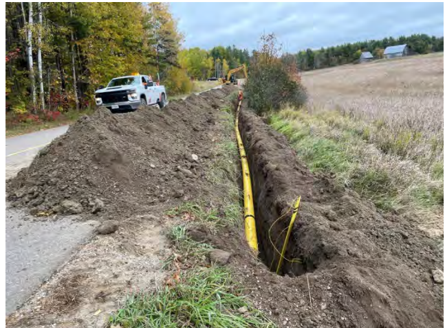
Photo 6: Pipeline stringing activities on Mcgaghan Road (October 15, 2024).
