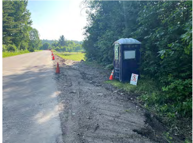
Photo 40: Regraded and back-filled ROW on Mcgaghran Road (June 30, 2025).
