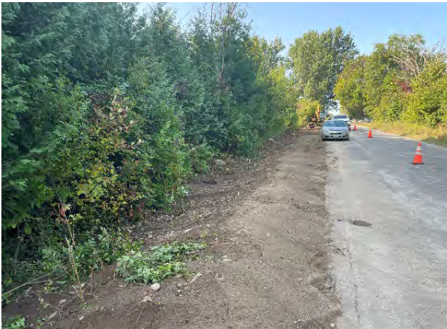
Photo 53: Restoration completed on Mcgaghran Road, east of Bulger Road (September 9, 2025).
