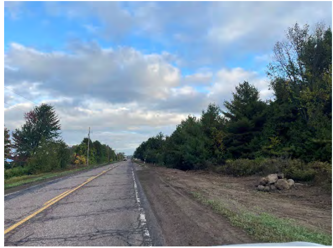
Photo 56: Restoration completed on Bulger Road (September 24, 2025).
