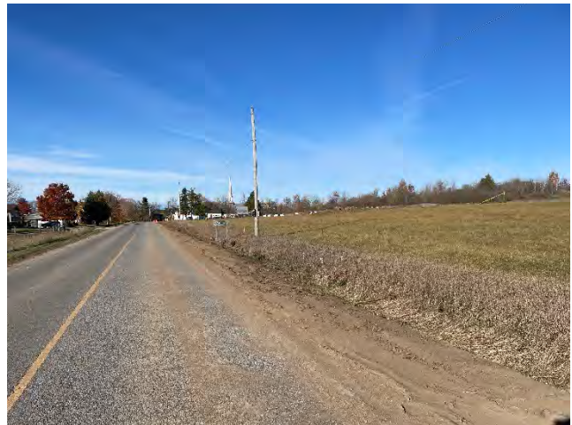
Photo 10: Restoration completed on Micksburg Road, west of McGuinty Road (October 28, 2024).
