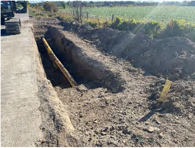
Photo 55: Tie-in on Mcgaghran Road, east of Pine Valley Road (September 19, 2025).
