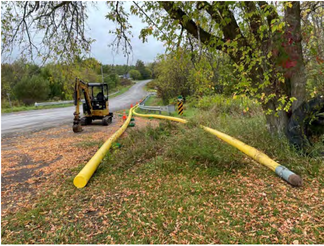
Photo 1: Pipeline stringing activities on Micksburg Road ROW. (September 23, 2024).
