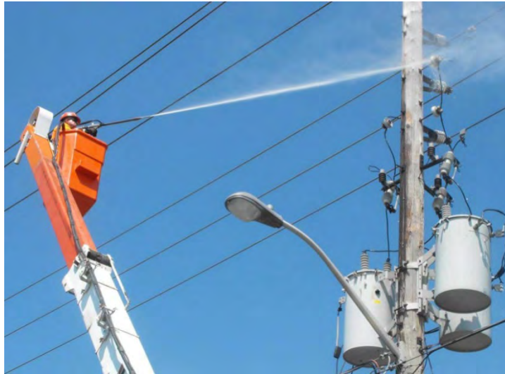
1 Figure 3: Insulator Washing in Progress
