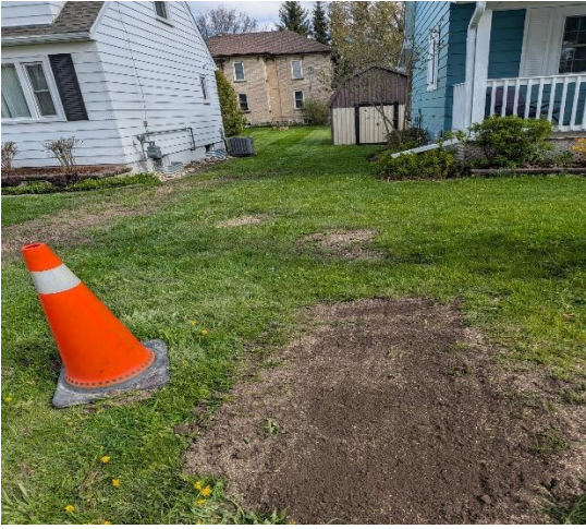
Photo 13: Restoration now completed at 115 William Street
