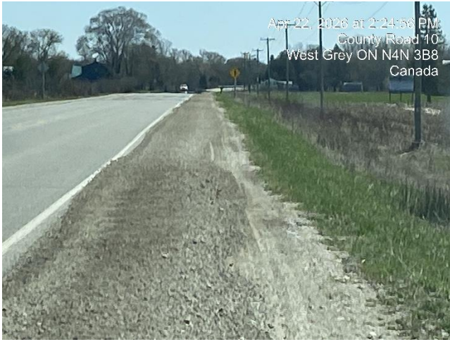
Photo 1: Reestablished shoulder of County Road 10
