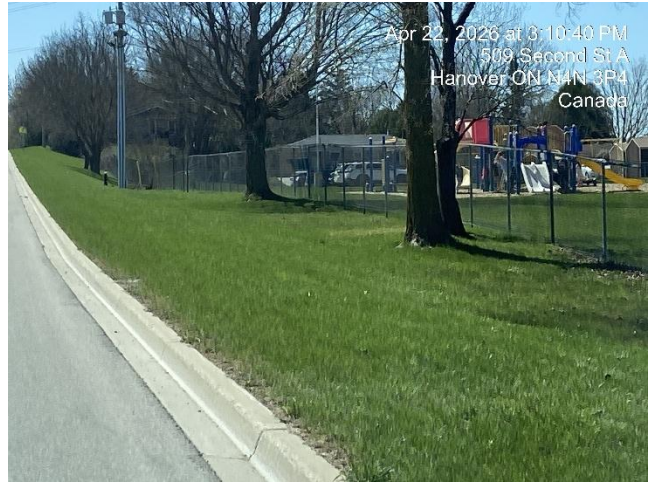
Photo 8: Restored road boulevard on Second Street in Hanover
