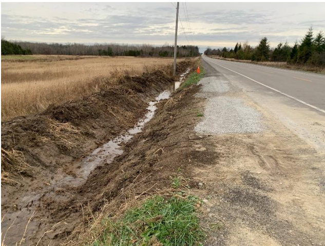
Photo 9: Reclaimed embankment along Sanford Road at the end of construction (November 14, 2024).
