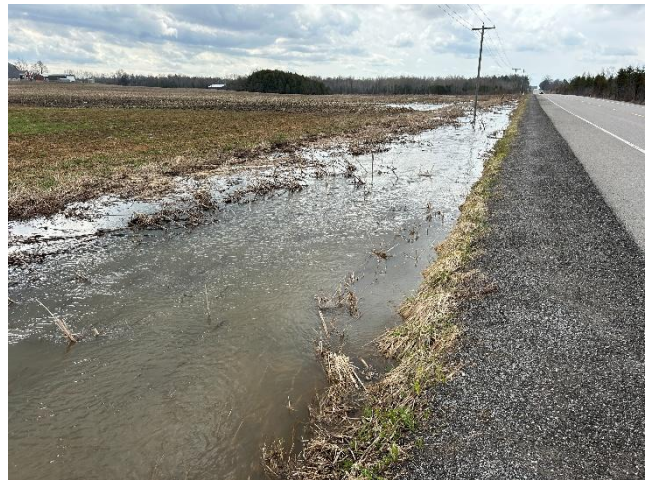
Photo 10: Current conditions of water flowing through stabilized embankment along Sanford Road (April 14, 2026).
