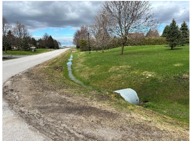
Photo 28: Current conditions of reclaimed road ditch along Lundy Drive (April 14, 2026).
