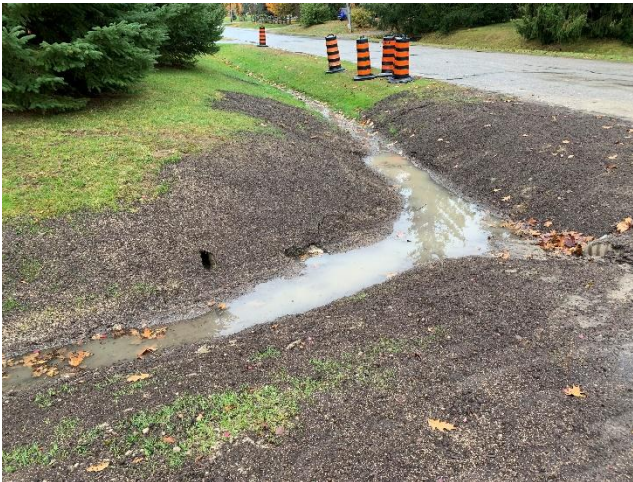
Photo 23: Water ponding after restoration at the corner of Smith Drive and James Place in the Village of Sanford (October 29, 2024).
