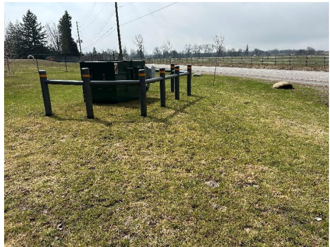
Photo 4: ROW condition in 2026 of Photo 3 around the upgraded station at the southeast Corner of Bolton Road and Concession 6 (April 14, 2026).
