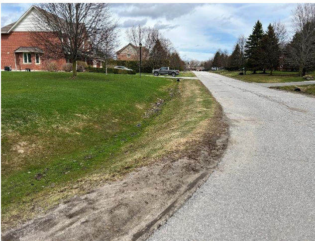
Photo 29: Current condition of reclaimed road ditch within the Village of Sanford (April 14, 2026).
