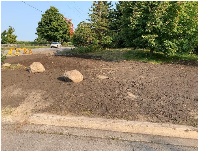
Photo 1: Restoration completed at the northeast corner of Bolton Road and Concession 6 at the end of construction (September 13, 2024).
